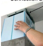
Assembling bracket hole on the Ceiling Connection Sheet
