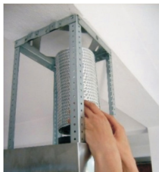
Installation bracket channels on ceiling mounting plate
