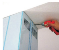
Assembling bracket hole on the Ceiling Connection Sheet
